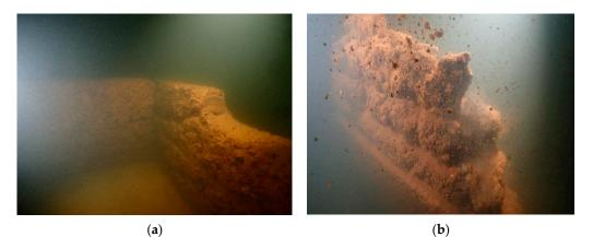
**Figure 54.** Walls of enclosed compounds, which were built with rammed earth. (**a**) more compact. (**b**) less compact.
