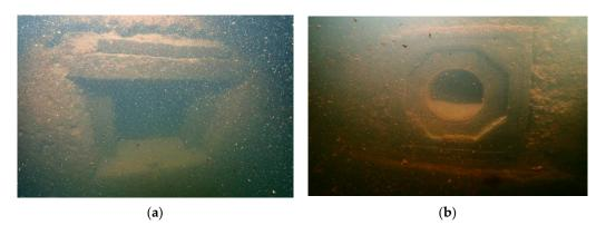
Figure 57. Square (a) and round (b) dog holes in the lower part of a wall of a sijiaolou building.
