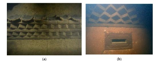
**Figure 55.** (**a**) The gray sand wall of a sijiaolou building. (**b**) Defensive gun-holes on the wall of a sijiaolou building.
