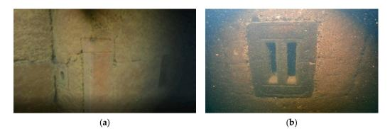
**Figure 56.** The solid wall structure of a sijiaolou building constructed with rammed gray sand. (**a**) on the corner of the wall. (**b**) in the middle of the wall.
