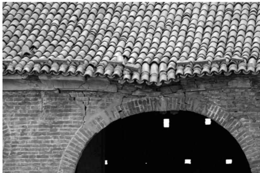
**Figure 10.** Sliding collapse of a brick arch.
