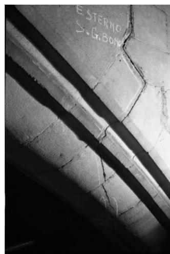
**Figure 3.** Shear/tension failure of masonry arch, Milan Cathedral (1965). At exterior arch from Pier 43 to Pier 44 on Figure 4.
