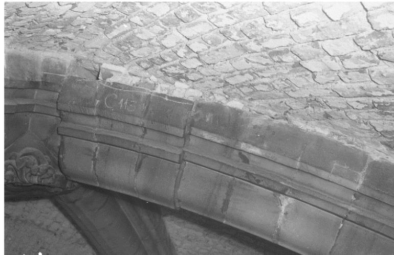
**Figure 6.** Sliding failure of a vault rib from Milan Cathedral (1965). Vault 113 in the plan in Figure 4.
